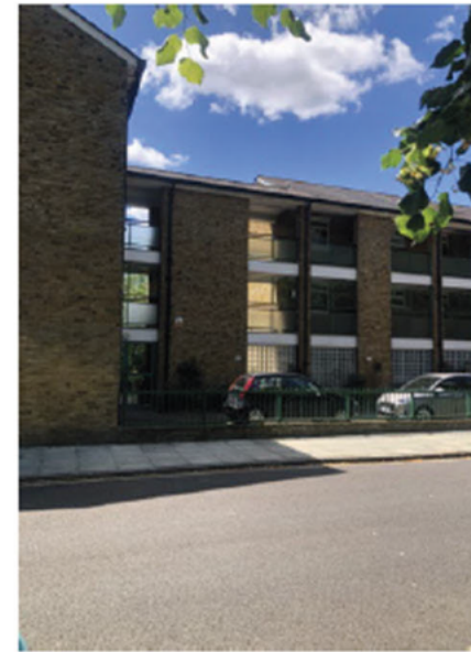
03. View through to the courtyard
