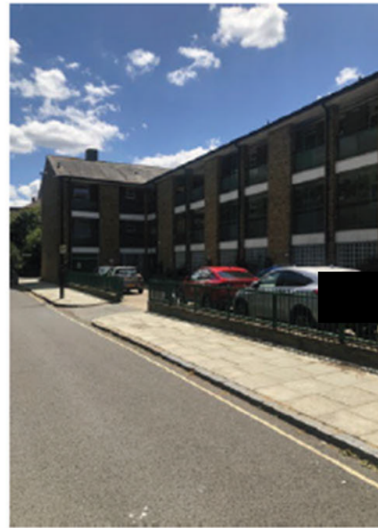
02. View along Flinton Street
