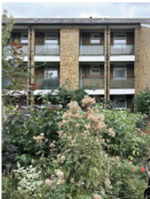
01. Deck access from courtyard garden
